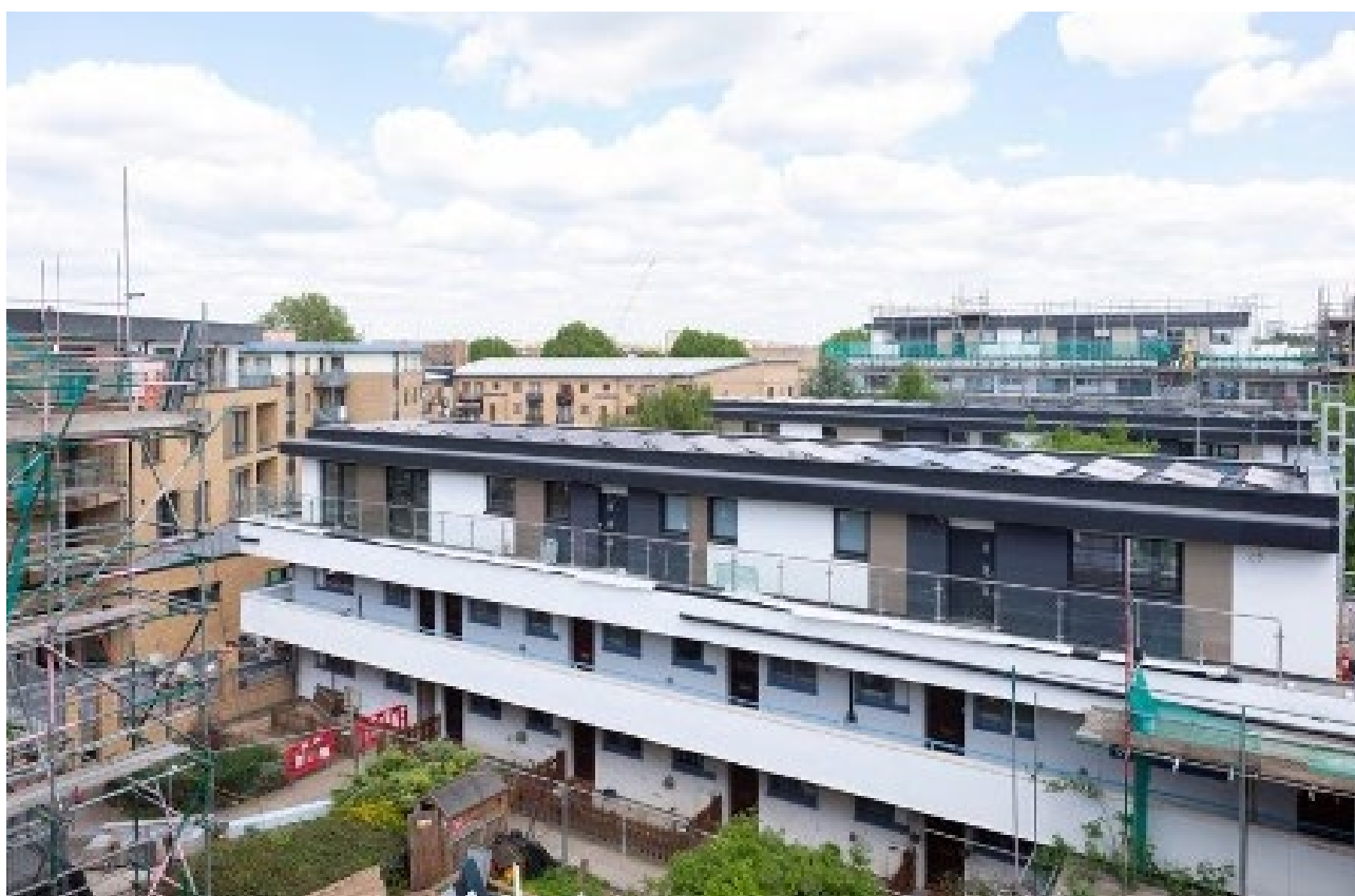
Waltherton and Elgin Community Homes, community-led scheme that builds new social rent homes through roof extensions, which also include the installation of solar panels. Photo source: WECH's website.
